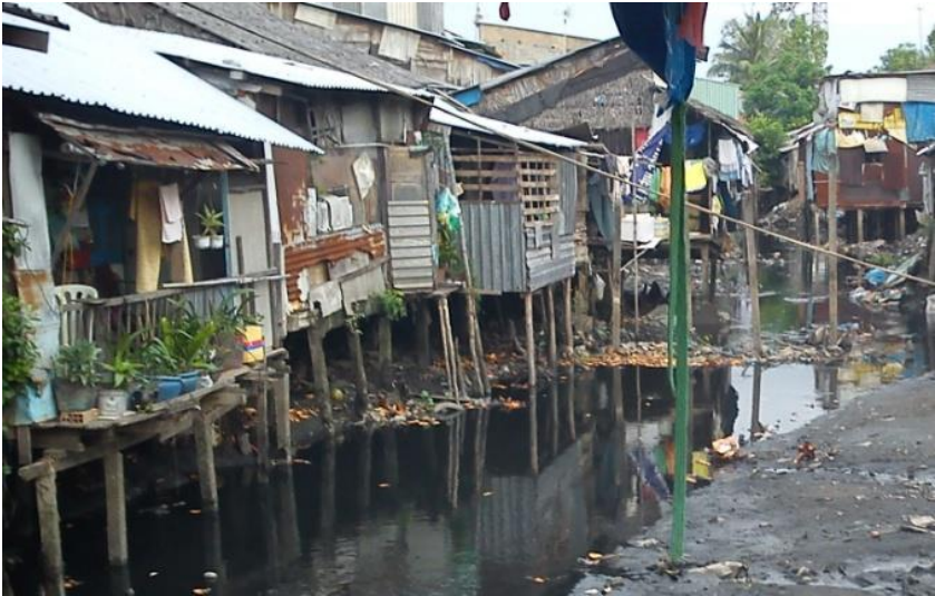
Figure 38: “Floating houses” constructed at the edge of canals in urban Ninh Kieu district (source: Panagiota Kotsila)
